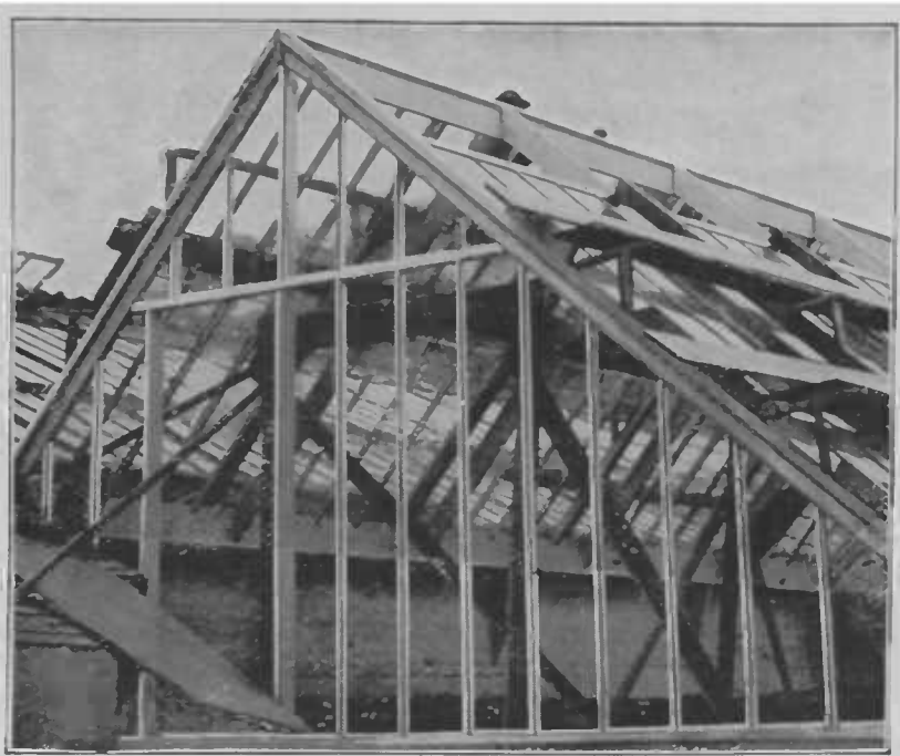
11. Construction of a rafter-and-sash bar frame.
